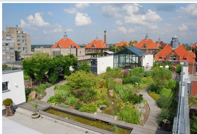
Green roof over a clinic in Berlin 3
