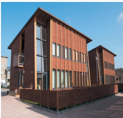
Low-rise apartment buildings, Eco-District Viikki, Finland iii
